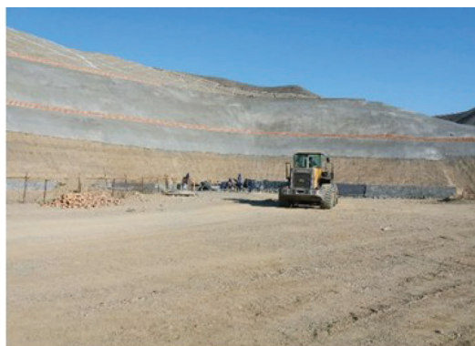
Preliminary Excavation of Pit
