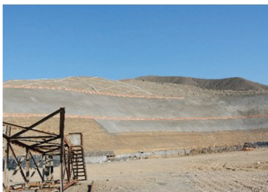
Side-slope Protection Construction
